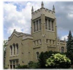
Yorkminster Park Baptist Church in Toronto.
