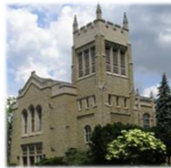
Yorkminster Park Baptist Church in Toronto.
