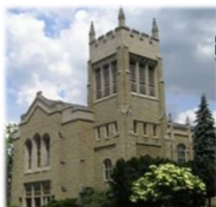
Yorkminster Park Baptist Church in Toronto.
