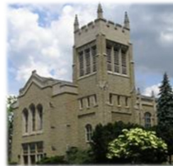
Yorkminster Park Baptist Church in Toronto.
