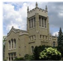
Yorkminster Park Baptist Church in Toronto.
